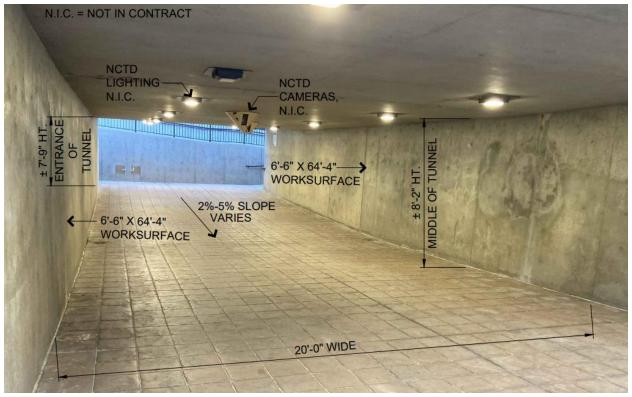
Sidewall view of pedestrian tunnel ramps (Artist encouraged to include artwork on both the west and east entry-way walls):
